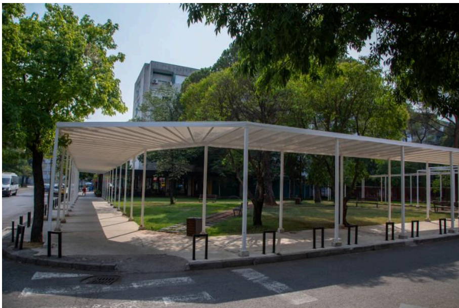
Figure 6: Location neat elementary school after introduction of weather protecting canopy making school entrance approachable and enhancing walkability of the area
