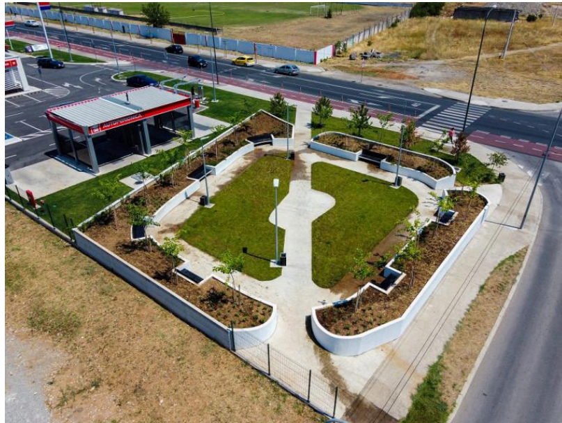
Figure 9: Mikro 020 solution, previously neglected urban pocket greened and formed into a Park of Energy. The intervention funded by the adjoining petrol station
